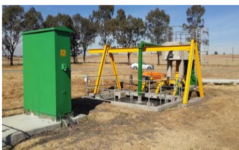
KINROSS SEWER PUMP STATION and WWTP
