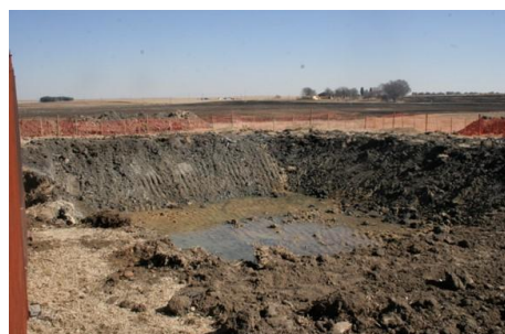
FIRST STREET SEWER PUMP STATION(EMERGENCY DAMS)
